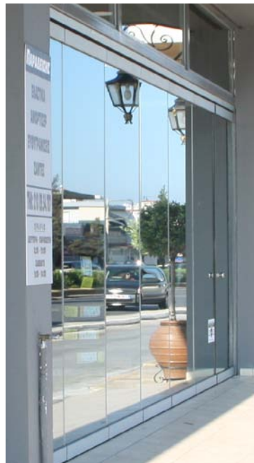
A minimal solution for a movable facade
